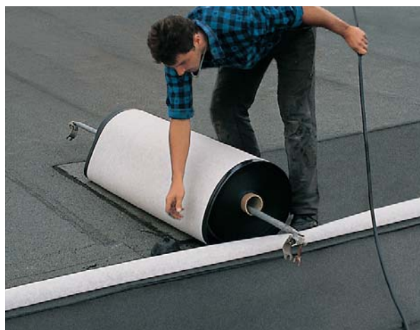
The back side of the NOVOPROOF® roof sealing sheet DA-S is furnished with a robust strong-fleece lamination.
