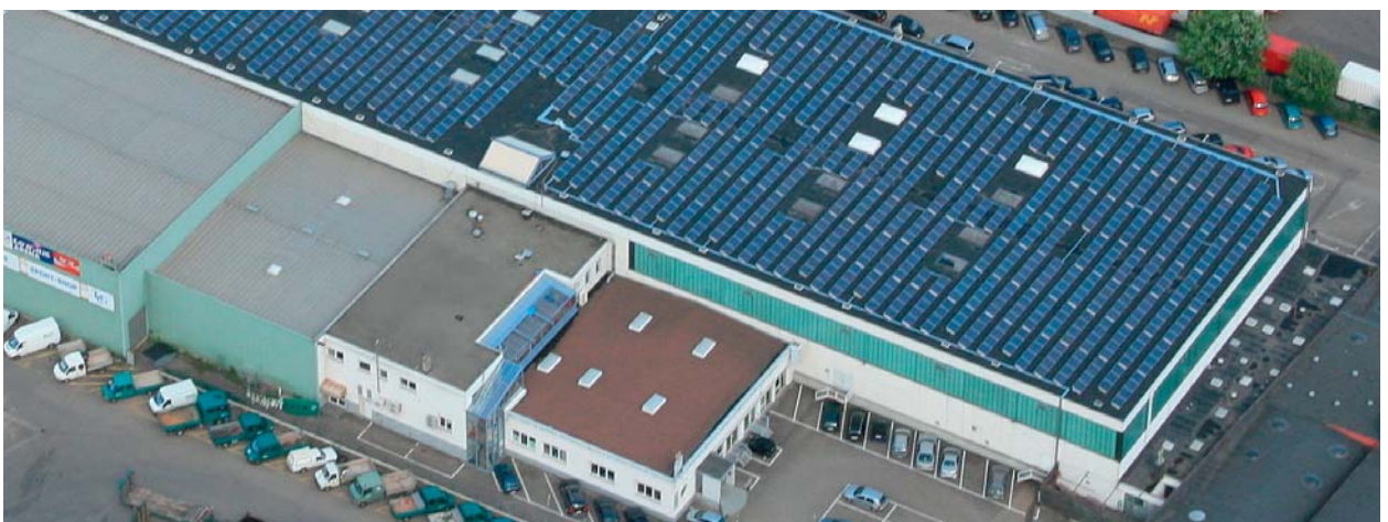
Solar system with 319 Kw total output on 10,000 m 2 EPDM roof sealing sheets NOVOPROOF® DA-K.
