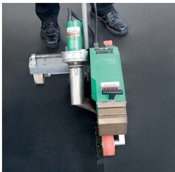
For the application on site: Hot-air welding with the welding machine.
