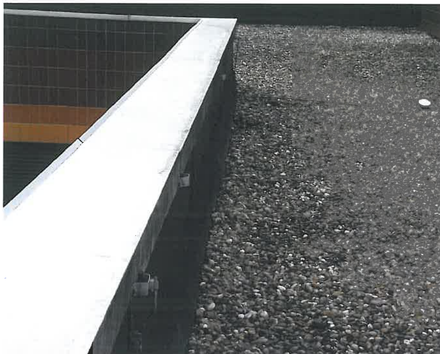
Fig. 5: General photograph of the roof parapet of the Training Centre Building at Wadern after 30 years in place; no signs of shrinkage stresses
