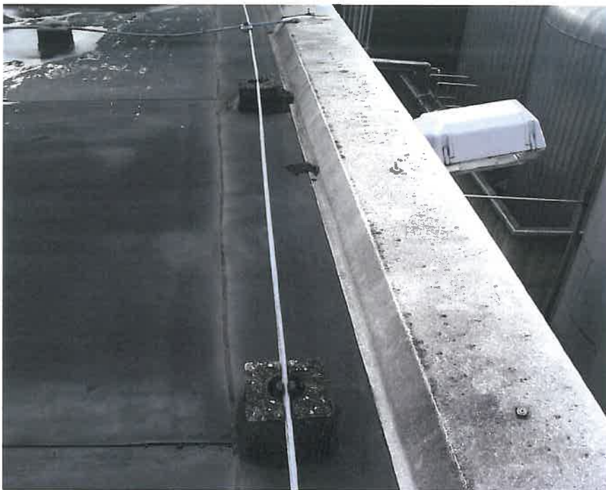
Fig. 2: General photograph of the roof parapet of the Karlsberg Brewery building at Homburg after 28 years in place; only slight signs of shrinkage stresses
