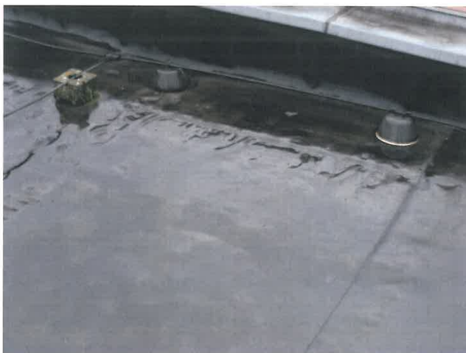
Fig 6: General photograph of the roof parapet of Saar Gummi hall 22 after 36 years in place; no signs of shrinkage stresses
