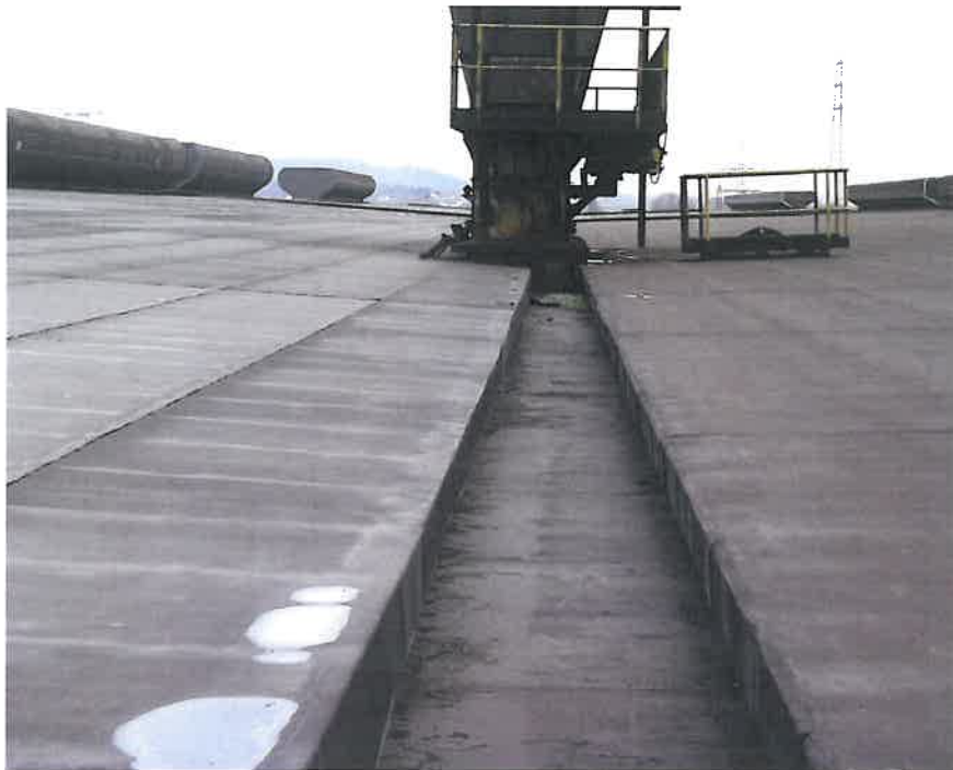
Fig. 1: General photograph of the channel of the Dillinger Hütte building after 29 years in place; no signs of shrinkage stresses
