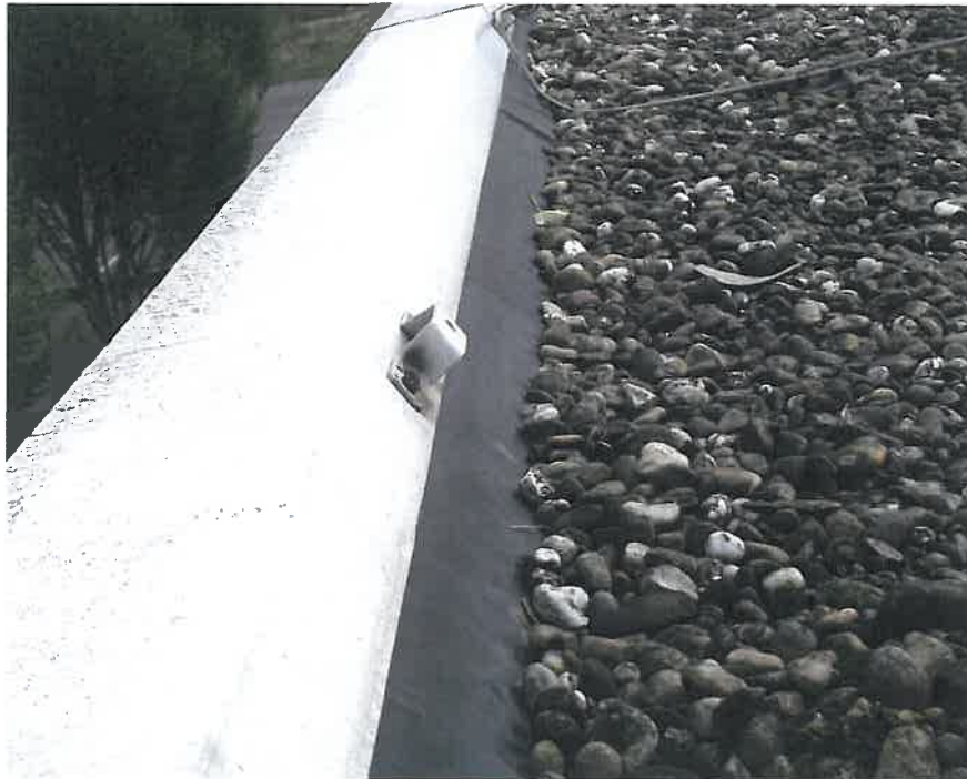
Fig. 3: General photograph of the roof parapet of the Swimming Baths Building at Wadern after 30 years in place; no signs of shrinkage stresses
