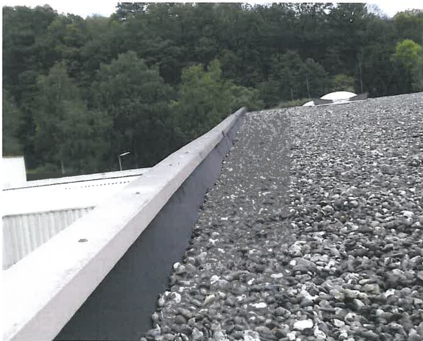
Fig. 4: General photograph of the roof parapet of the Army Building at Primstal after 27 years in place; no signs of shrinkage stresses
