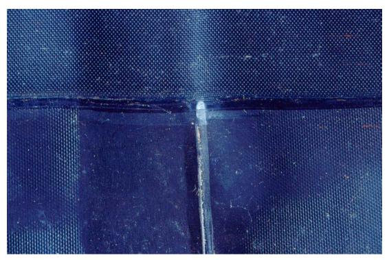
Figure 4: Sheet surface with T joint
