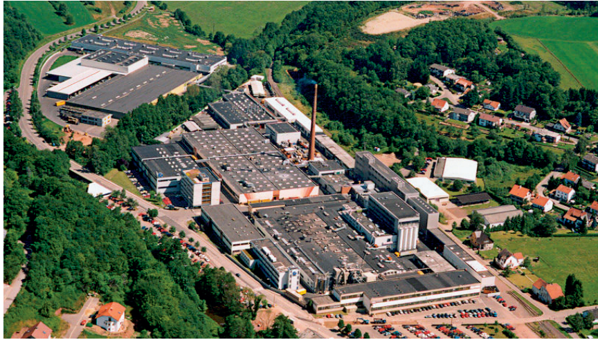
Company plant DURAPROOF technologies GmbH
