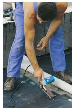
Sanding after weathering
