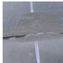
Prepared lap seam
