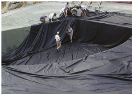
NOVOPROOF® TE as sealing membrane in a water treatment basin
