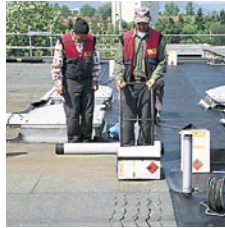
Application of adhesive
